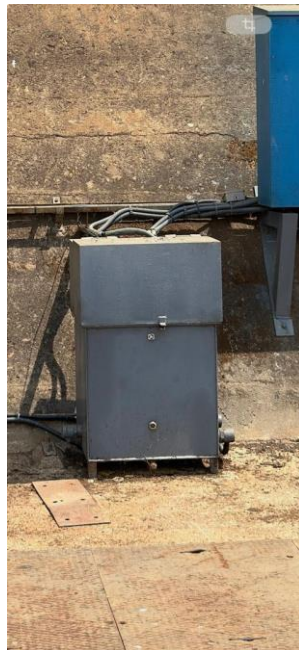
Figure 3: Centrale hydraulique
